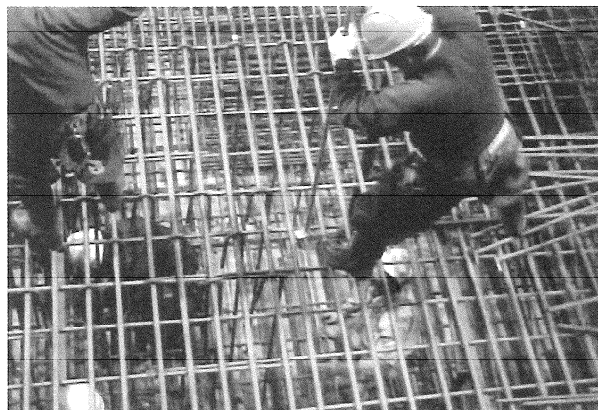
(b)底版の施工
